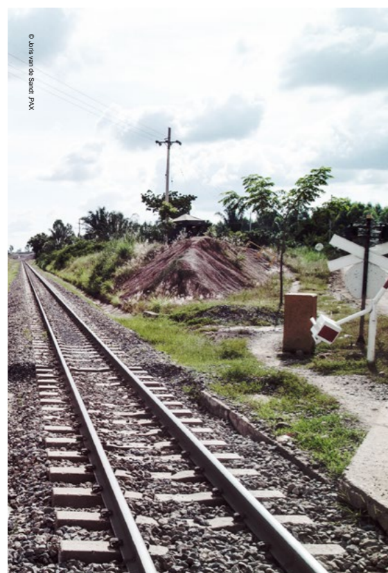
Guarded railway for coal transport to the coast.
