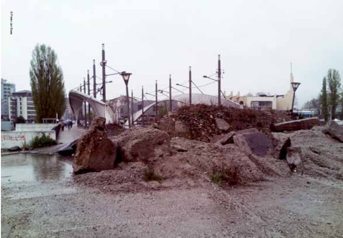
The barricade on the main bridge in Mitrovica is a reminder of the segregation with which people in Mitrovica have lived for 14 years.
