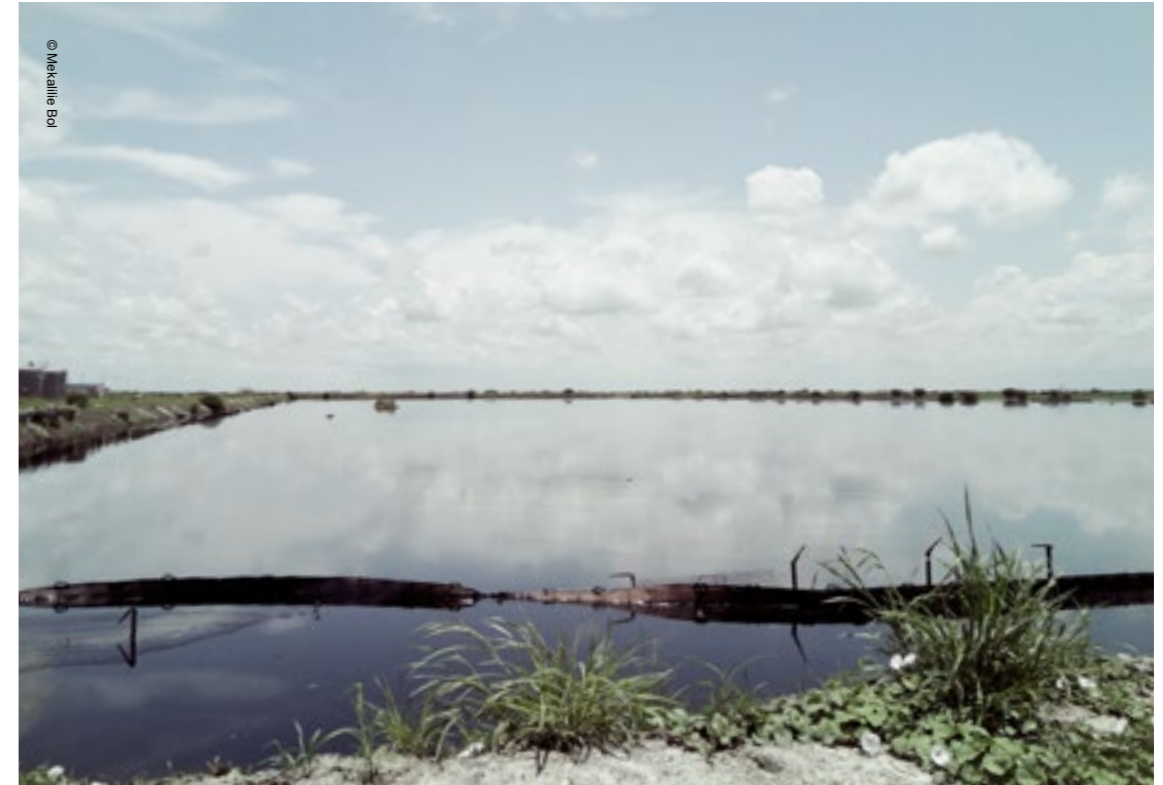
PDOC waste water basin insufficiently lined posing danger to the environment, 2011
